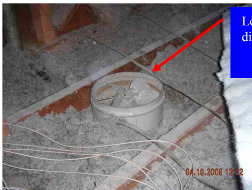
Kitchen exhaust fan discharge to cabinet
