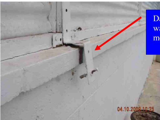
Paint deterioration
