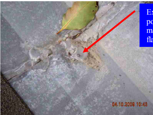
Plastic waste pipes passing through garage fire-rated ceiling finish
