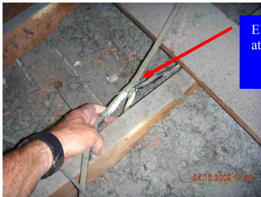
Abandoned wiring at crawl space
