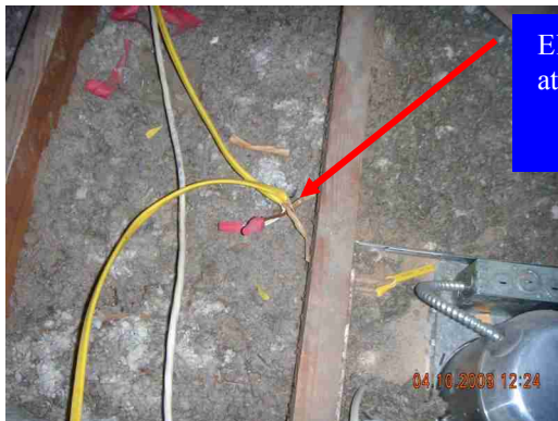
Electrical splice at attic
